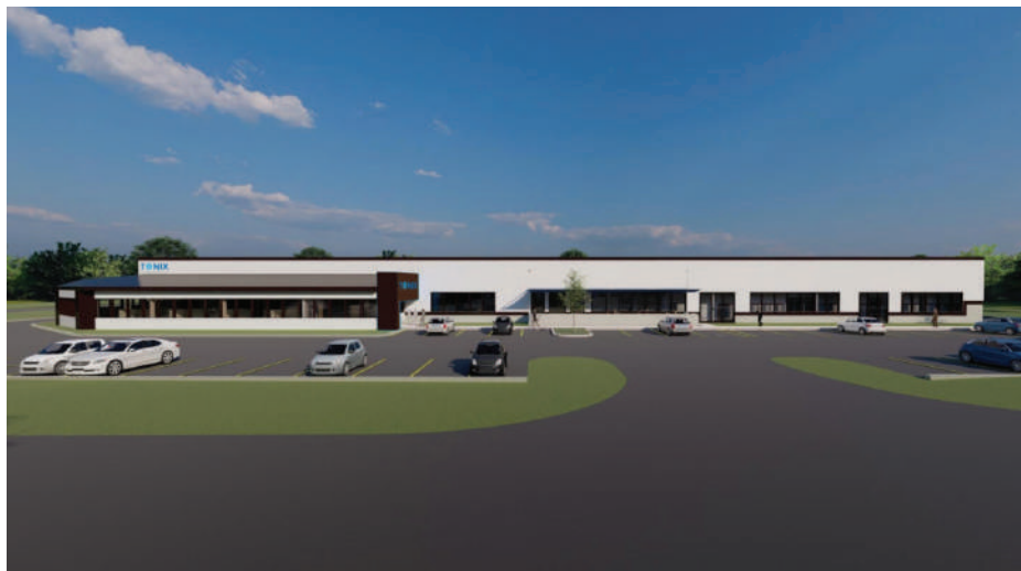
PREFAB ADDITION Site work is underway for a vaccine manufacturing facility in Massachusetts.
