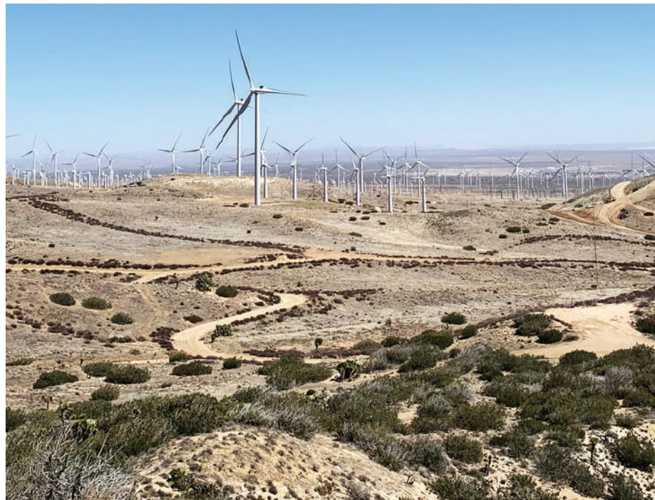
REVAMP Mortenson will replace 60 1-MW turbines with 17 3-MW turbines for Terra-Gen in California.
